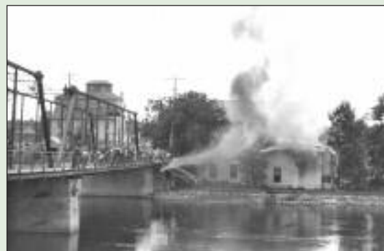
Mattress factory next to Whipple Truss Bridge (Gail Corbett photo)
