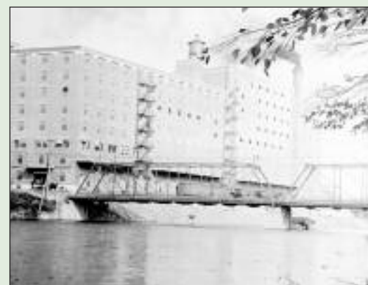
Whipple Truss Bridge, P.C.M.A. photo (1979-010)
